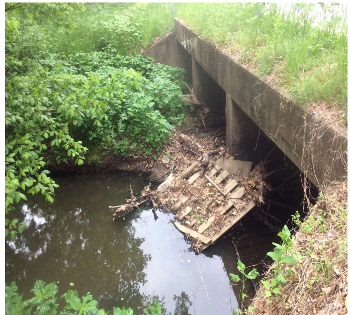
PHOTO 2 Description Channel right side. Debris and silt
