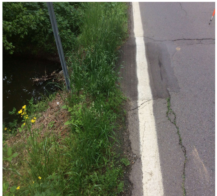
PHOTO 2 Description Roadway - Barrel 3 right: Settlement at pavement edge
